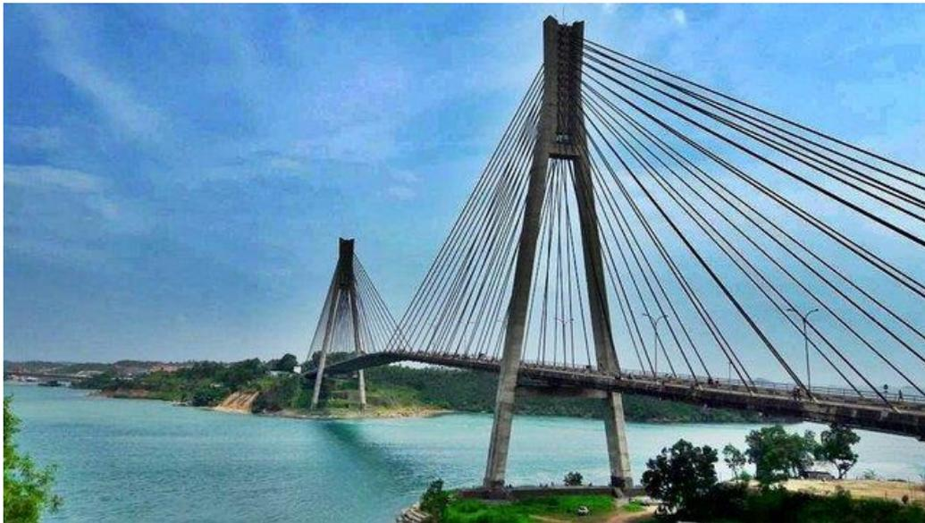
Gambar 1. *Cable Stayed Bridge* (Jembatan Kabel Penahan/kabel tetap)
